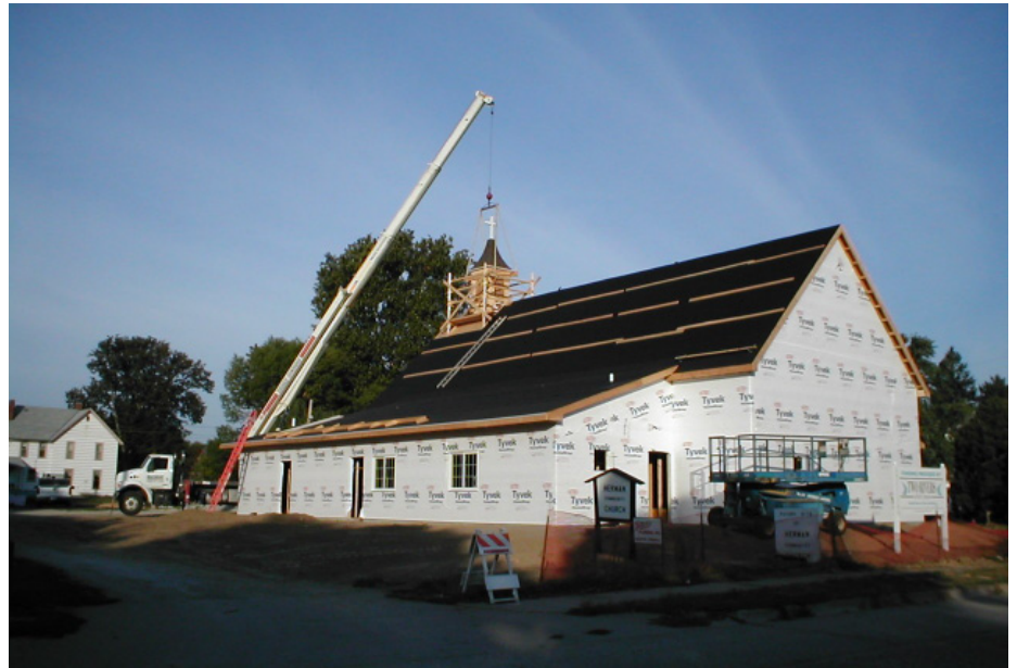
Setting the bell tower at Herman Community Church.
